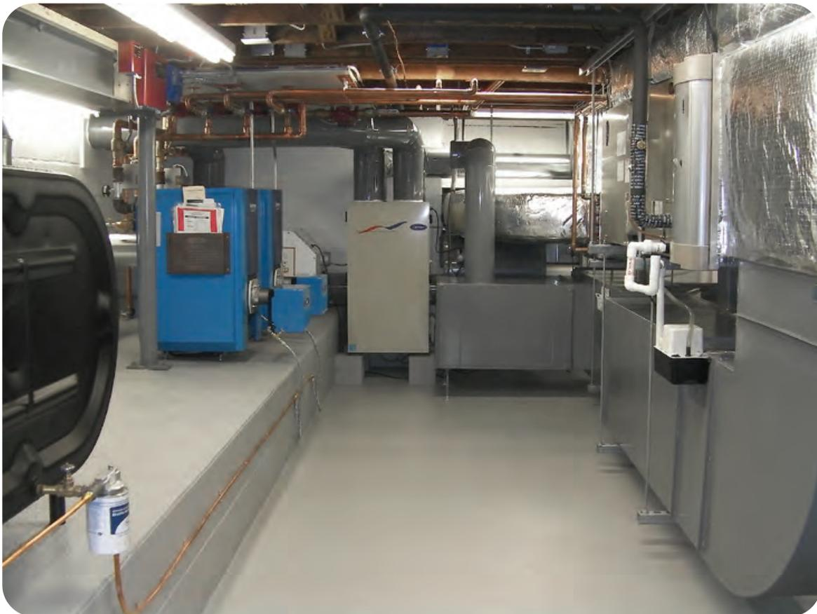
Once the cellar space was deconstructed and made a-new, I had the opportunity to do my best work. Viewing from 6-o'clock, clockwise – the equipment: oil tanks; twin Buderus boilers; Santa Fe dehumidifier; Carrier HRV; Carrier air handler.
