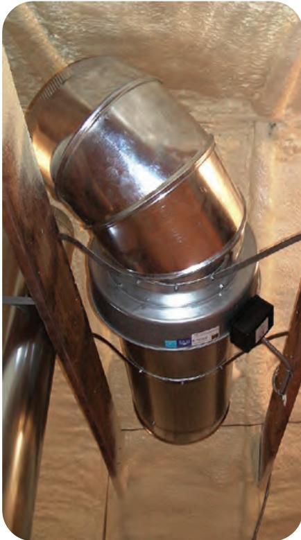
A 900-CFM attic exhaust fan was installed and vented through the roof (see page 13)– this acts as a whole-house fan and removes insulation “out-gas” odors from the attic.
