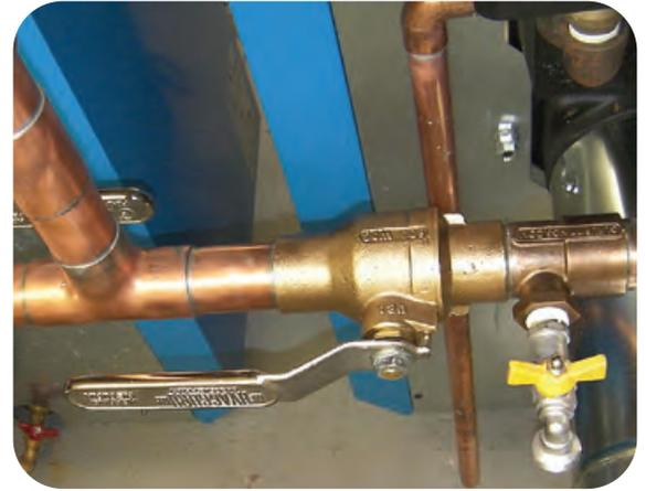
Like my bronze flanges, the 1-1/2" Male (Street) X 1-1/2" Female X 1/2" IPS lead-free, bronze sweat (solderable) Tee eliminates the need for a length of copper pipe to join it to a valve or fitting.
