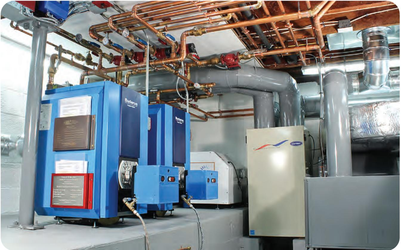
My document holder and valve handle inventions can be seen on the boiler and local piping. The Buderus cast iron boilers are oil-fired G215/3 models, and are controlled by a Tekmar staging/temperature modulation control.
