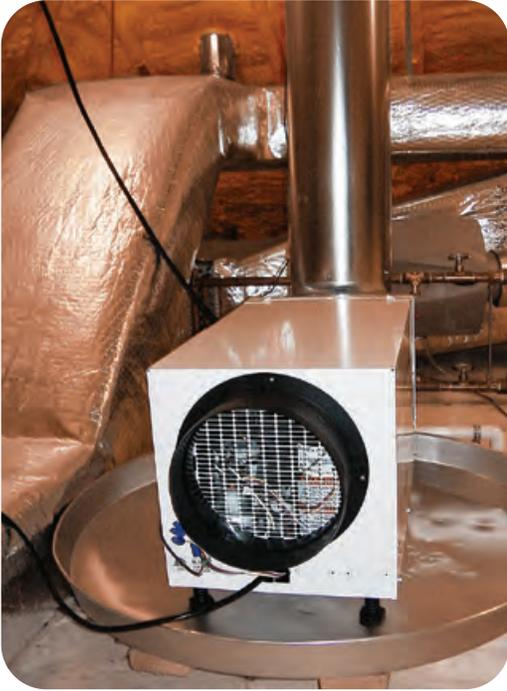
Closed-cell foam insulation (sprayed directly onto the underside of the roof) acts as a vapor barrier. Therefore, a dehumidifier was required to manage relative humidity in the attic, via a hard-wired de-humidistat.
