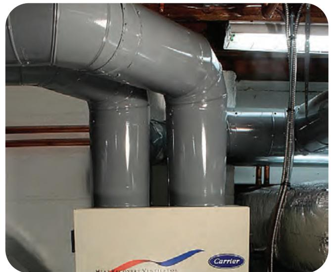
Carrier Heat Recovery Ventilator (HRV) ties into the 1<sup>st</sup> floor A/H duct system and provides fresh air supply/stale air exhaust.
