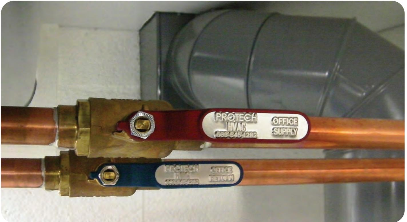
Nickel-plated handle inserts were customized to remove all mystery from the aspect of the heating system the valves (and pipes) serve. These plate inserts are pressed into place after the handles are installed, ensuring that the text is always upright regardless of valve installation direction.
