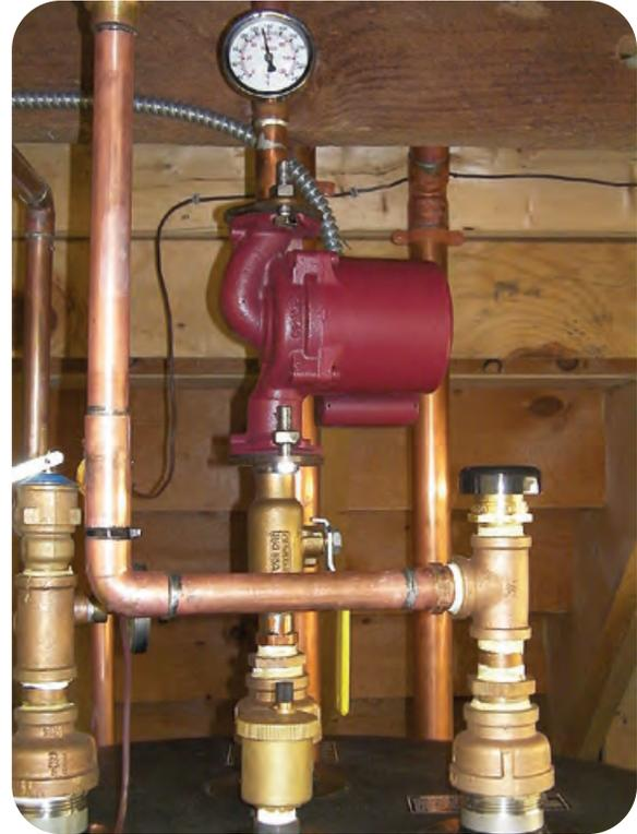
Triangle Tube lifetime-warranty, stainless steel indirect-fired water heater (left). My lead-free bronze circulator flanges connect to the Grundfos circulator for hot water re-circulation. Potable water connections (right) are on top, and boiler water connections (not shown) are in the back of the tank-within-a-tank.
