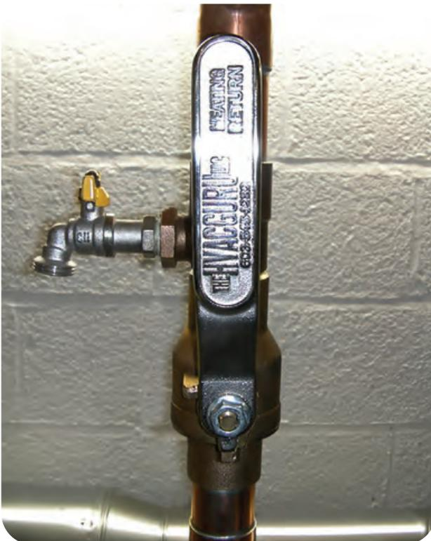
Tee is behind the nickel-plated, polished/buffed bronze 1-1/2" valve handle, and has a purge valve (yellow handle) attached.
