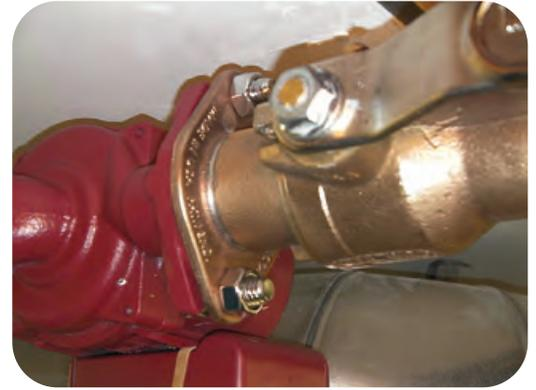
Bronze ITS-Flanges clean up nicely with a wire wheel and complimentary stainless steel, or chrome-plated, nuts and bolts add form and corrosion resistance. Solder flows evenly around the circumference of the flange for a perfect seal.
