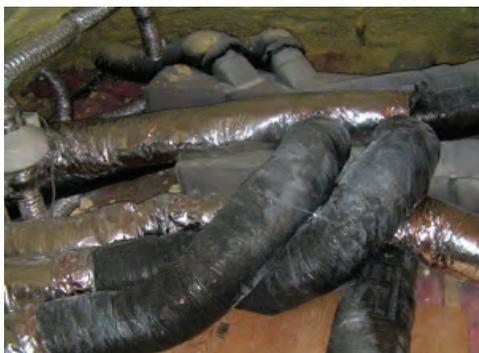
All of the “run-outs” in the attic were flex duct, and were kinked and excessively long. Consequently, many of the rooms below were starved for sufficient airflow. The flex ducts were installed so haphazardly that most were crushed over time by people stepping on them.
