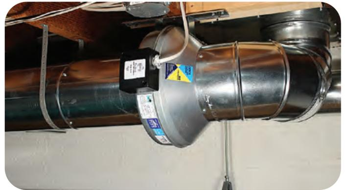
Two 600-CFM exhaust fans (identical to the master bath) for 1<sup>st</sup> floor baths were installed and vented through rim joists.
