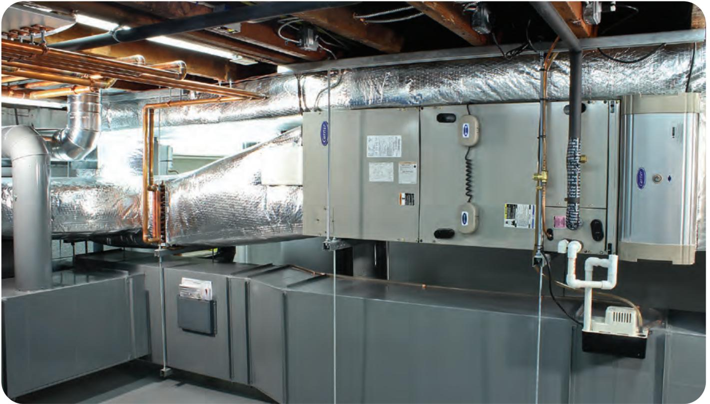
Carrier 5-ton Air Handler (A/H) – Valves on refrigerant lines; HEPA/electronic air filter; UV lights and WIFI-connected system control add effectiveness and utility to the hydro-air system. I designed all custom-fabricated ducts to minimize static pressure and maximize airflow efficiency and distribution effectiveness.
