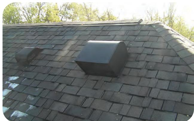
From top left, clockwise: 32-foot stainless steel Z-Flex chimney liner passes up through existing chimney; close-up of termination; whole house fan vent and master bath exhaust vent.
