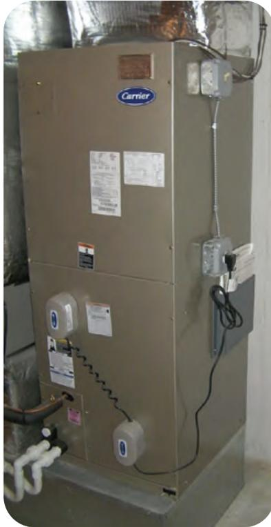
This 2-½ ton A/H was added to heat and cool a remote area of the 1<sup>st</sup> floor that always struggled to be heated and cooled satisfactorily. This system includes a bypass humidifier, dual UltraViolet lights and a combination electronic/High-Efficiency Particulate Air (HEPA) filter. My bronze plaque design (top right) and aluminum document holder (right side of A/H) add contact information and utility to the system.
