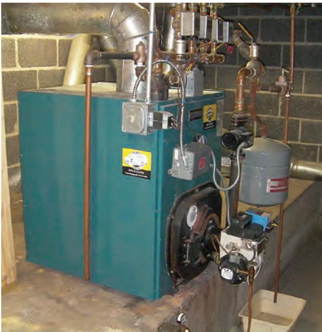
Each heating zone was controlled by a thermostat and zone valve. One circulator proved insufficient to supply hot boiler water to all zones simultaneously.
