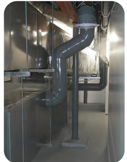
Painting ductwork added 16 hours of labor cost and \$200, plus or minus, of other direct/variable costs. The white diffuser (right image) delivers fresh air to the mechanical room. The same fresh air supply feeds the return plenum of the A/H.
