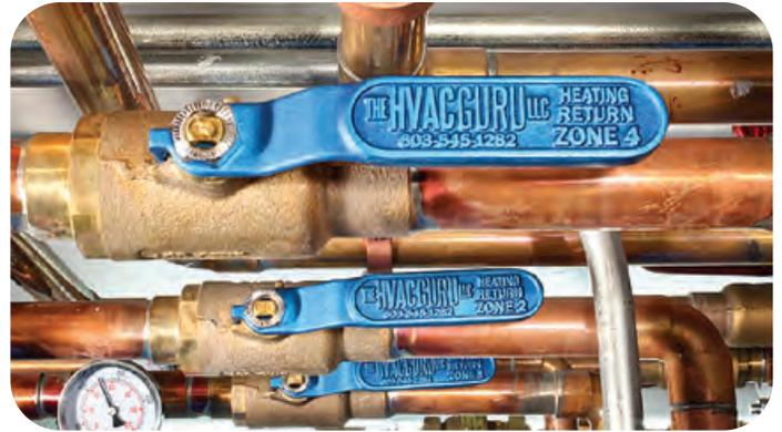
Red and blue anodized aluminum handles intuitively differentiate supply (hot) from return (cold) pipes.
