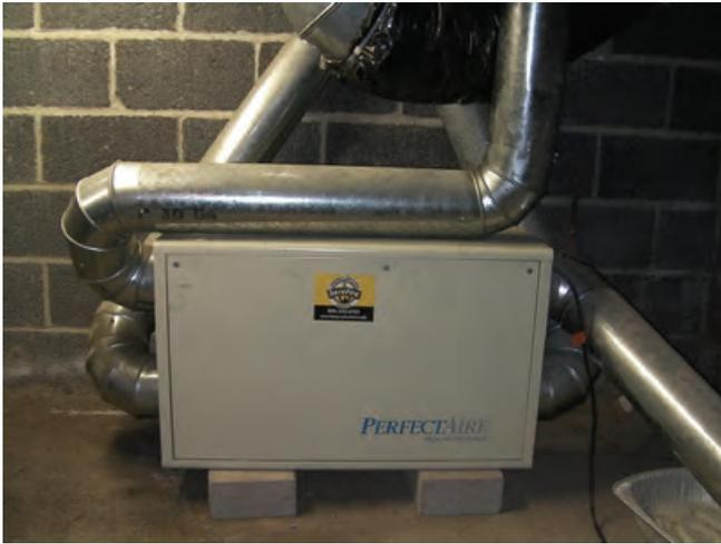
The HRV never functioned properly due to incorrect duct design and installation.
