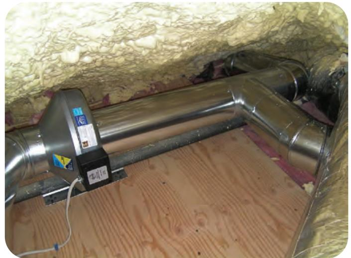
This 600 CFM fan removes air from 2 locations in the master bath and exhausts through the roof (see page 13).
